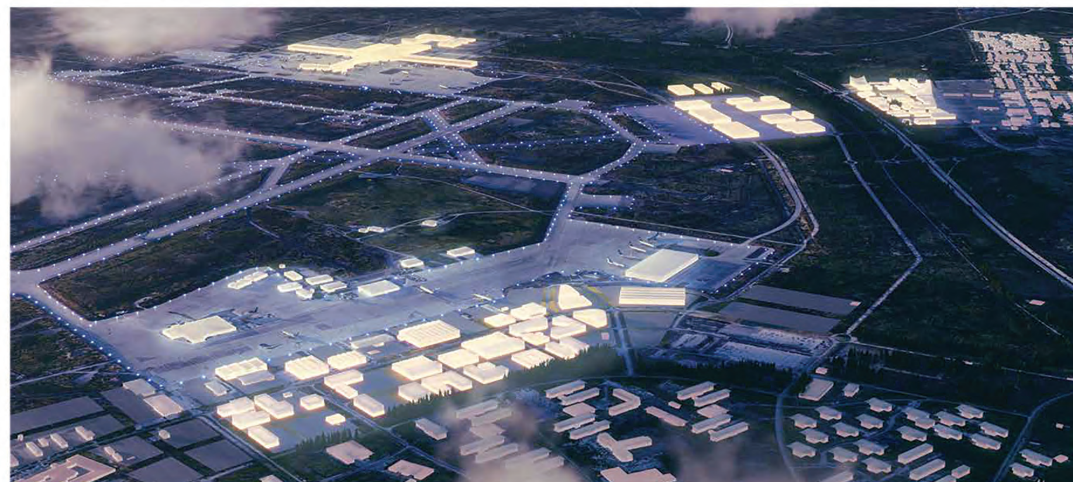
Northwest view of the Eco-Tech Park at Ásbrú Airside
